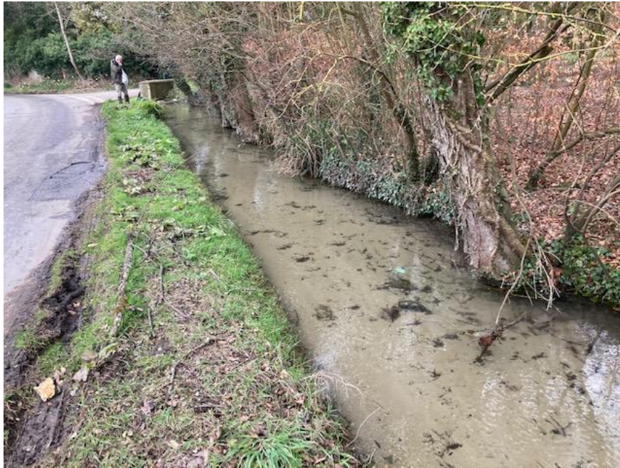
Figure 11: Accumulation of sand and fine sediment in an over-wide uniform section of channel
