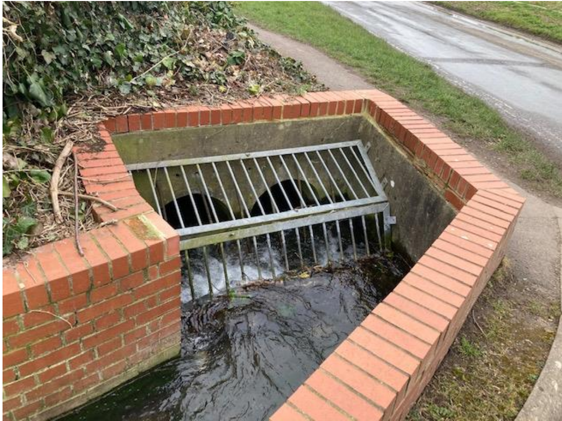
Figure 12: Twin pipes forming a culvert alongside the main Benson runway
