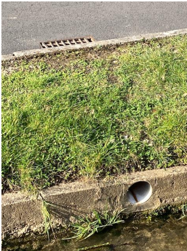
Figure 10: Road run-off piped directly into the stream
