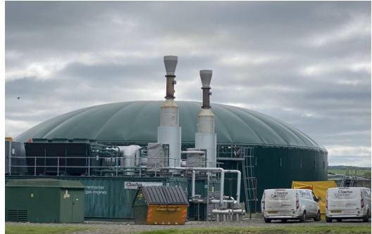
(Right) One of five green digesters behind two engines which burn the methane produced in the digesters to generate 2.4MW of electricity.
